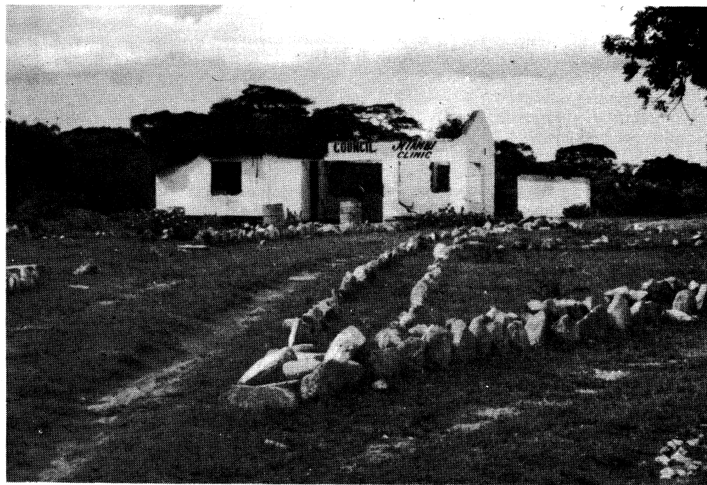
Living quarters in the bush — a bombed out clinic. The officer slept in the Maternity ward.
