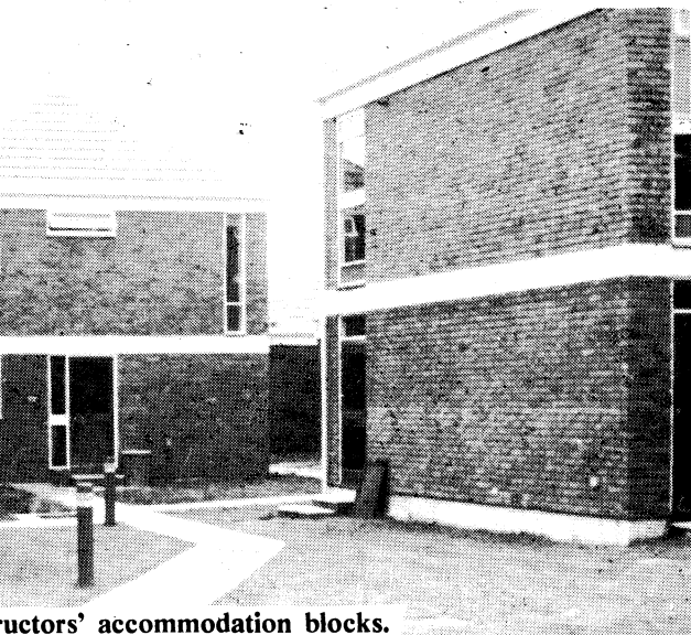
Instructors' accommodation blocks.
